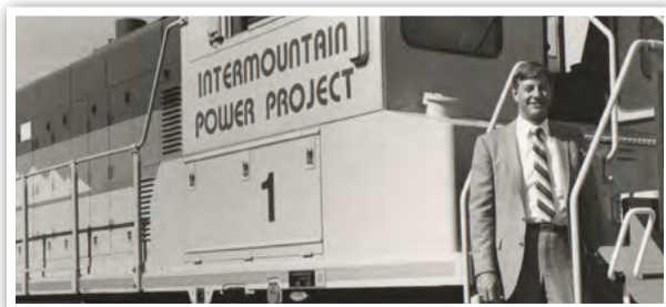
First coal train to arrive at the Project site.
